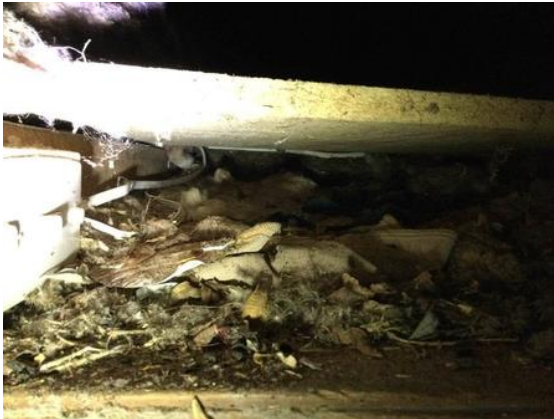
Some insulation missing in some areas
