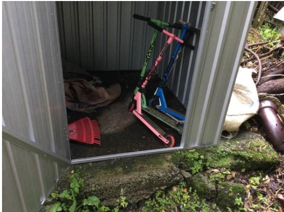
Shed has water visible on the ground
