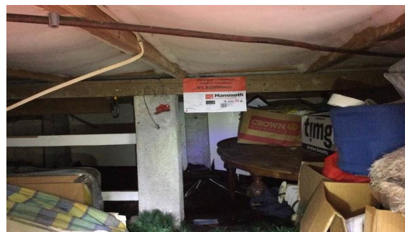
R1.9 insulation label underneath rear extension
