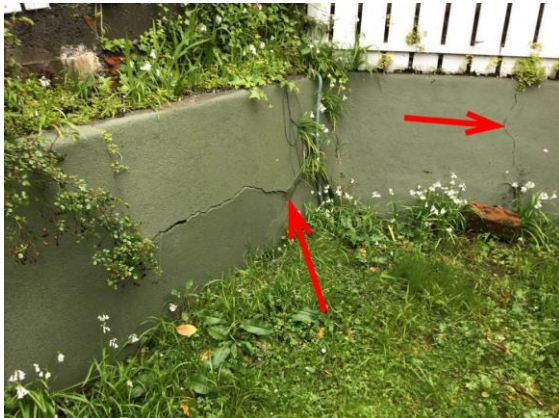
Visible cracks
