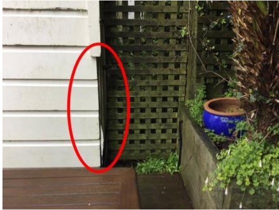
Missing cladding
