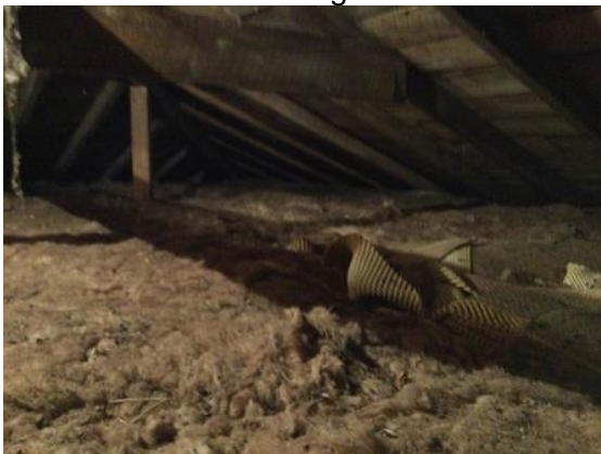
Some insulation missing in some areas
